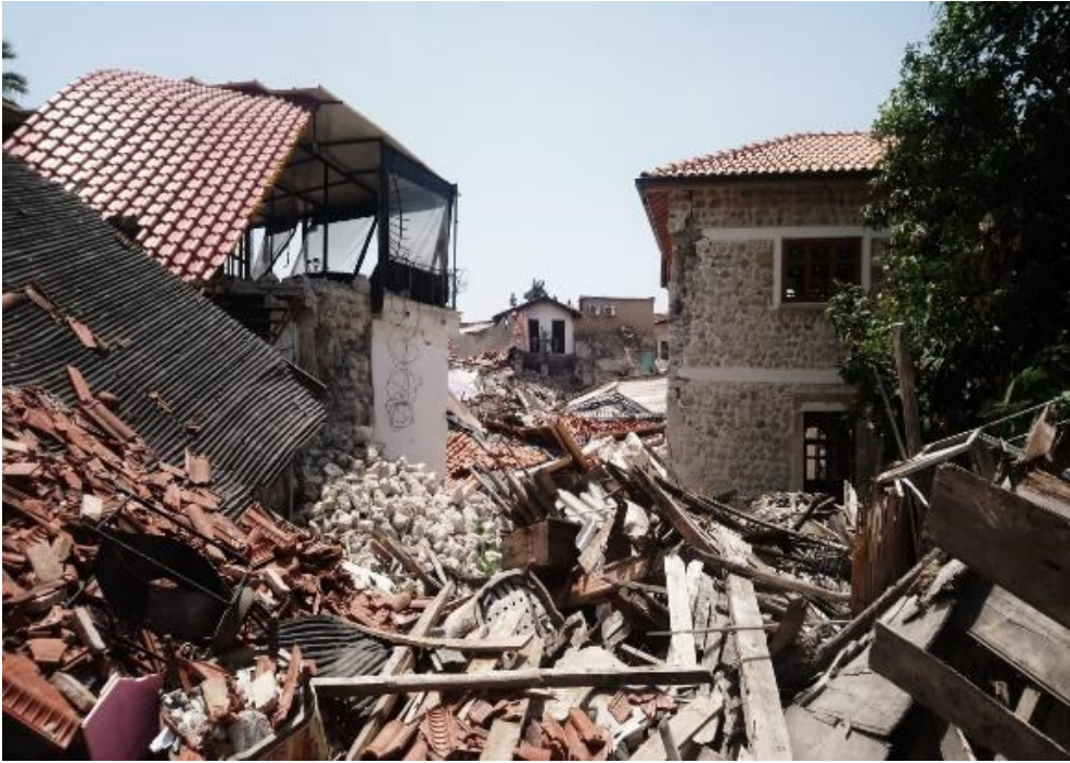
Photo 1. Demolished buildings in Old Antakya.
