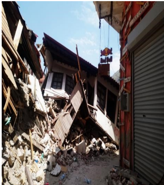
Photo 2 and 3. Rubble completely blocking the street in Old Antakya.
